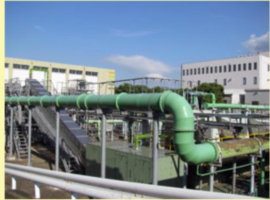
Hiagari Sewage Treatment Plant
